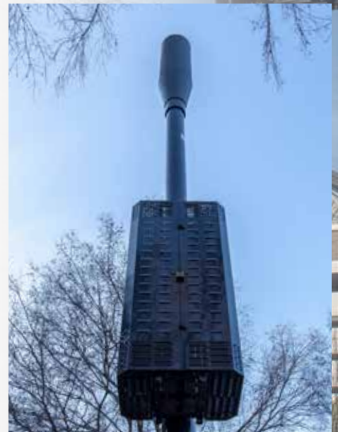
A recently installed small cell pole features an InvisiWave radome concealment for 5G mmWave radio/antennas, and a side mounted equipment shroud.
