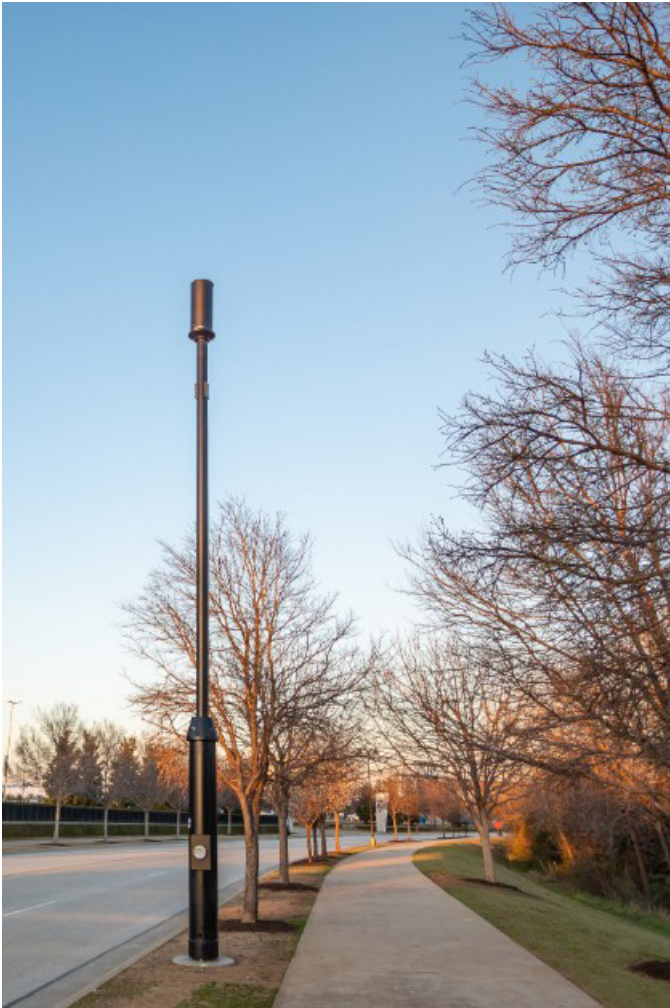
Figure 2: Integrated small cell pole combines and conceals all the elements needed for a complete 4G/5G small cell site.
