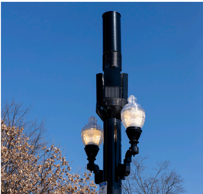
The small cell design includes variations to mount 4G antennas and 5G radios specific to each carrier at the top of the pole.
