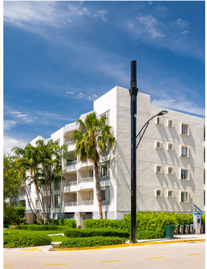
Figure 3. A small cell pole with 4G and 5G equipment installed in Miami Florida and customized to withstand windloads
