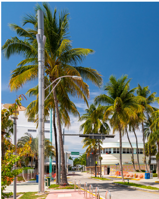
Figure 2. Raycap integrated small cell lightpole in Miami Florida
