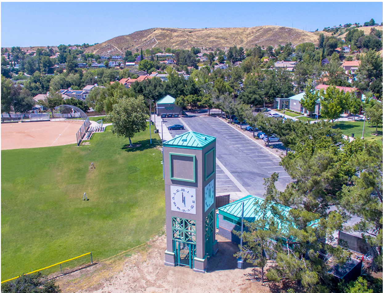
Figure 1. Example fully concealed macro cell site
