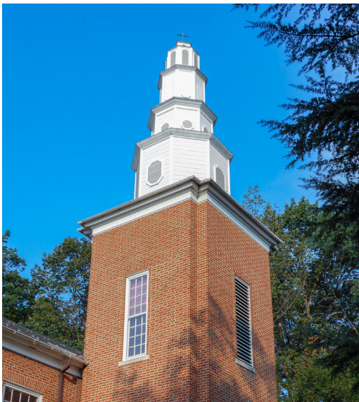
Figure 1: Virginia Steeple rebuilt to accommodate 5G equipment heat displacement.
