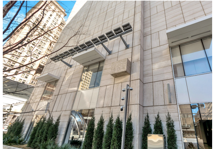
Figure 1 - A 5G small cell mounted on front of AT&T headquarters building
